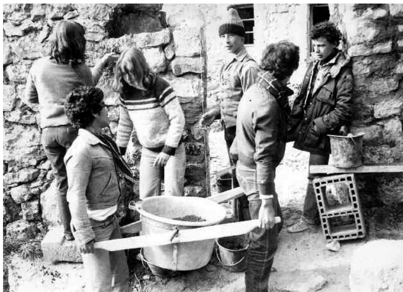
Transport de ciment
